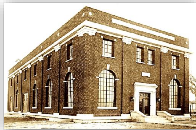
Montreal Tramway Power Plant
