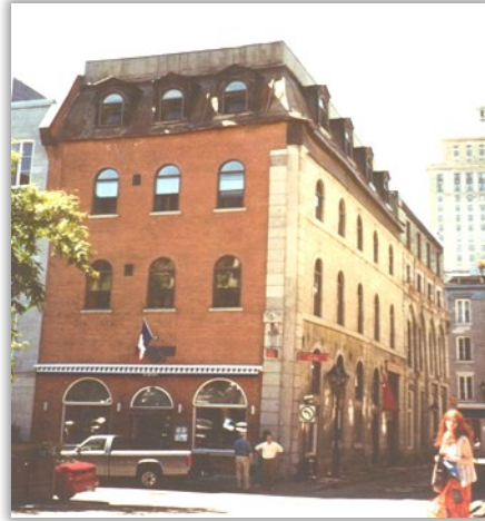
Archambault Building, 351 Place D'Youville, corner of Saint-Pierre Street.
