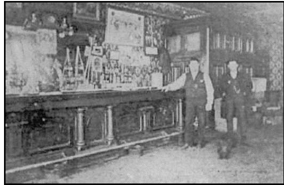
Interior of the saloon
