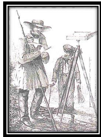
Aiming instrument for surveying circa 1830. A helper is carrying the famous chain.
